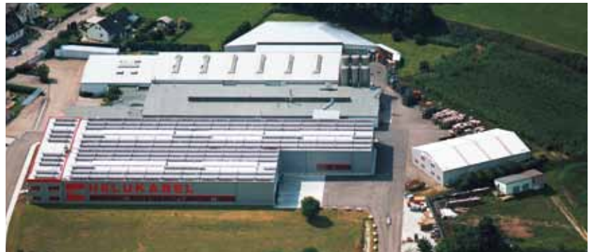
Production facility with a modern photovoltaic system, Windsbach / Germany
