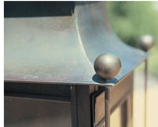
Heritage "clean" seams
