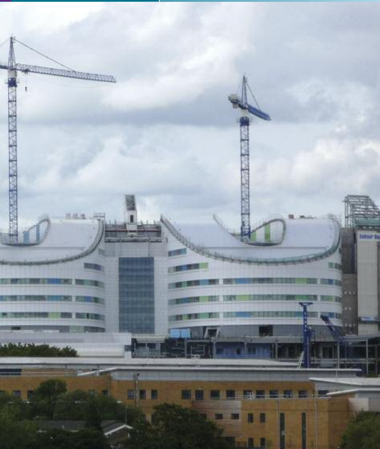
Queen Elizabeth Hospital, Birmingham Specification: Hattersley Thermal Balancing Valves
