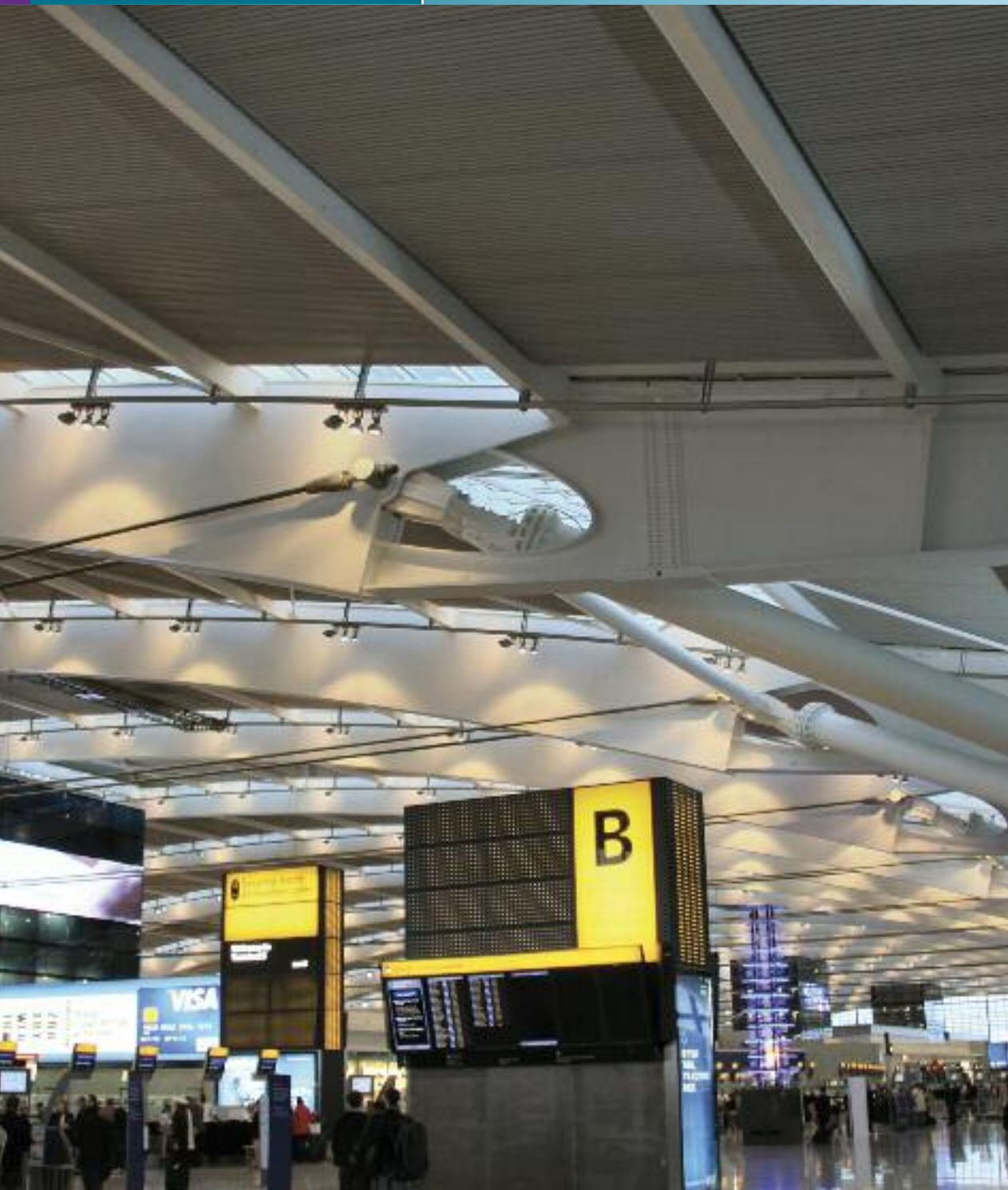
Terminal 5, Heathrow Airport, London Specification: Hattersley Automatic and Static Balancing Valves
