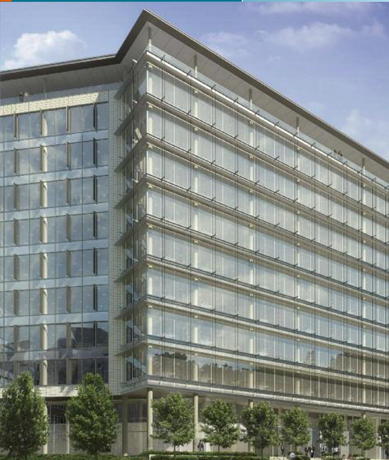
One Reading Central, Reading, Berkshire Specification: Hattersley Fixed Orifice Double Regulating Valves
