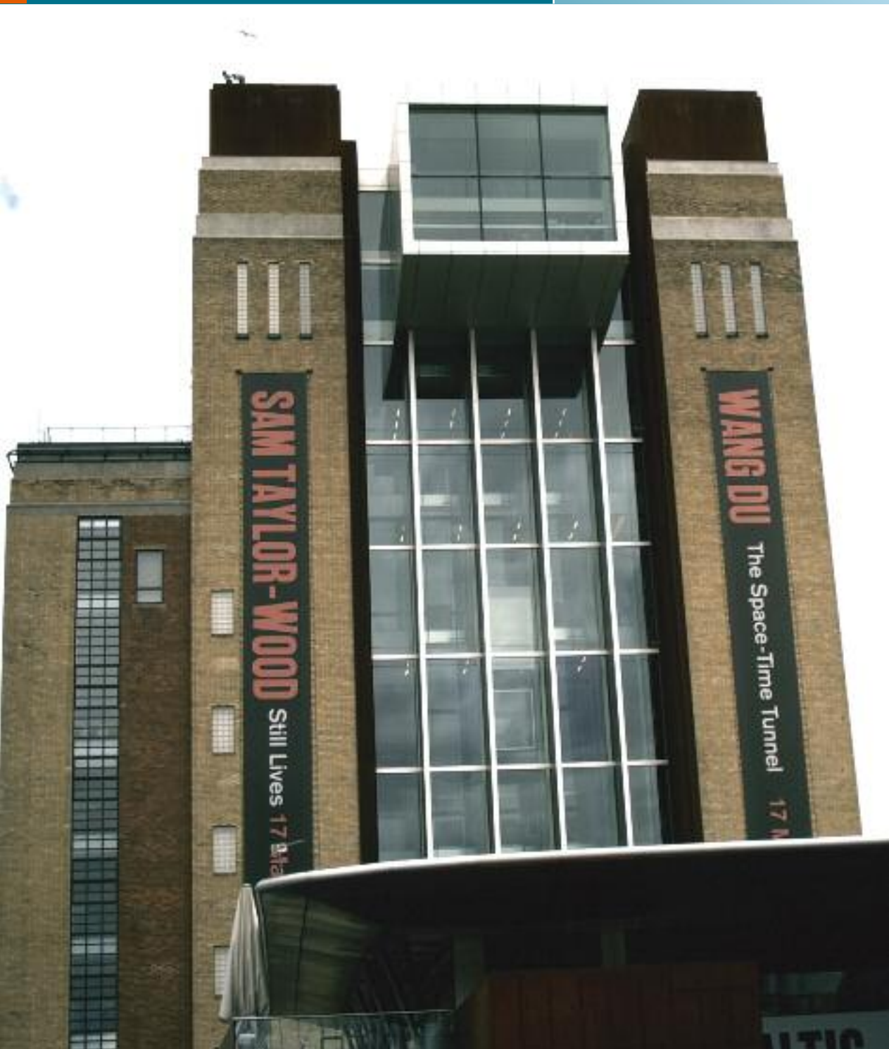
The Baltic Arts Centre, Gateshead, Tyne & Wear Specification: Range of Hattersley Commissioning and Traditional Valves
