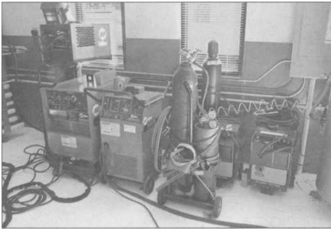
2.3 The welding corner of this well-equipped race-car prep shop holds a variety of equipment, from a large TIG machine at left (with cooling unit on top), to a heavy-duty plasma cutter, oxy-acetylene cutting/heating/welding outfit, and two small plasma cutters. Not shown here are the two MIG welders in use elsewhere in the shop.
