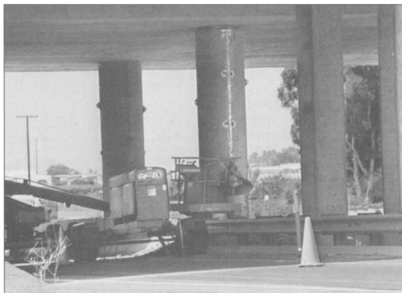
1.4 Under the center bridge column here are a welder (a machine) and a welder (a person). He is welding up steel enclosures for the concrete columns, to retrofit more strength in California bridges to meet newer earthquake codes.
