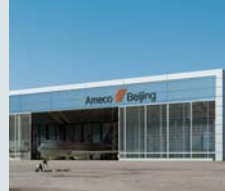
Ameco A380 Hangar, Beijing, China
