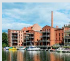
Studio flats, Brandenburg, Germany
