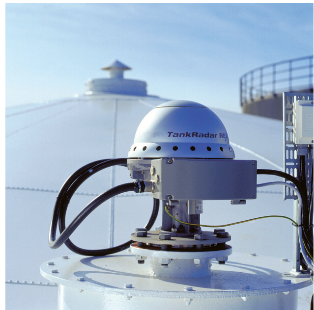
Rex gauges are installed using existing nozzles and manways.
