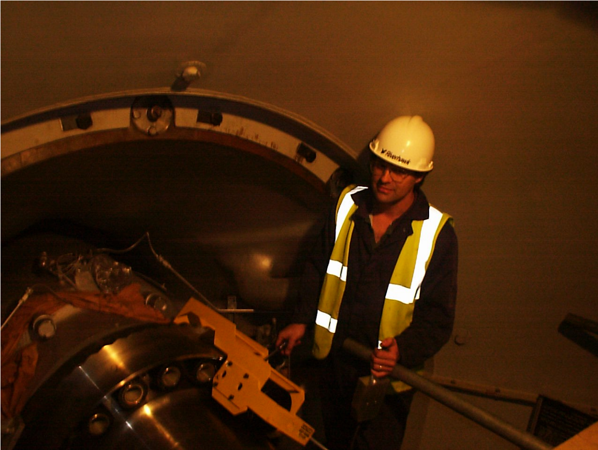
Photo 5 View of operator tightening nuts on Fr. 9FA turbine flange
