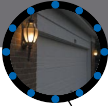
Garage lighting controls
