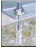
Fastening to Concrete with Threaded Rod
