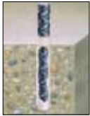
Doweling into Concrete with Rebar
