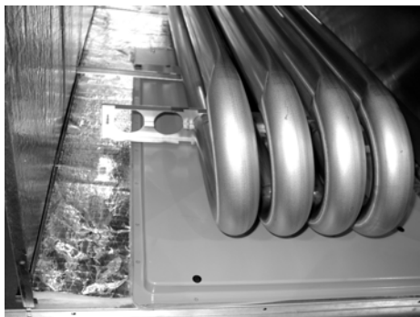
FIGURE 15 - DISCHARGE PANEL IN PLACE
