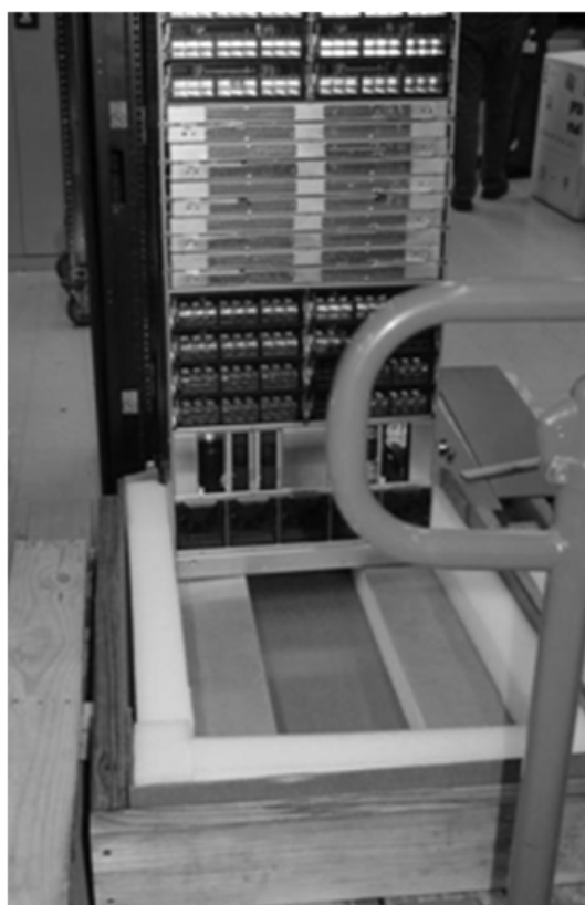
Figure 1-23 Sliding the Switch off the Pallet
