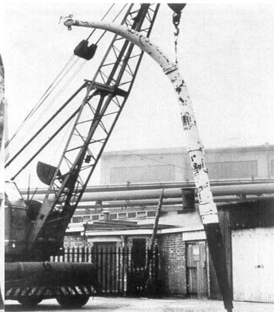
Figure 13: Complete S. S. Aquitania davit as delivered for inspection
