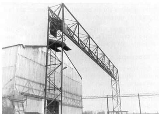
Figure 31: Valenciennes Works -General view of the loading portal before dismantling.
