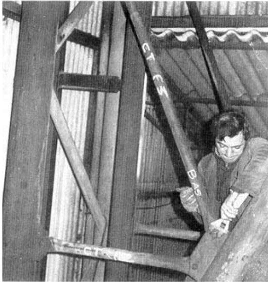
Figure 35: Dismantling of two bracing members with flattened ends.
