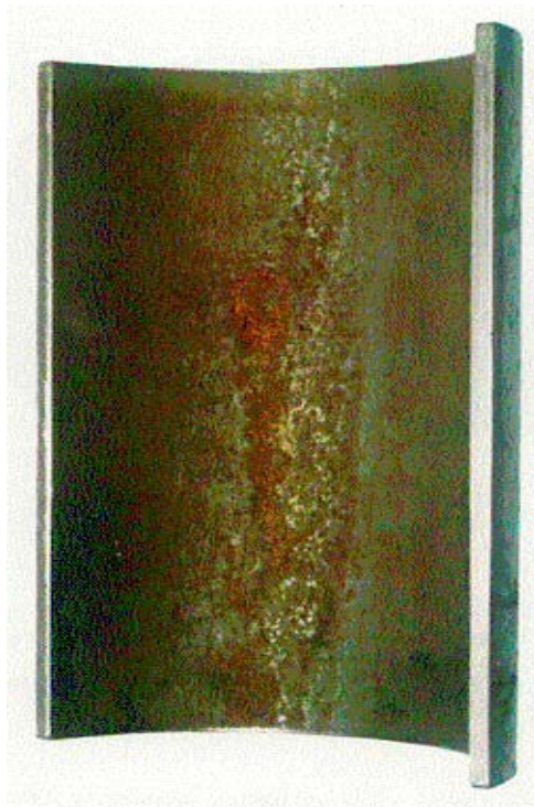
Figure 17: Circular hollow section 139.7 mm showing one of the half cylinders cut longitudinally. The slight amount of rust in the middle the tube is recent and has appeared since the tube was cut for inspection.
