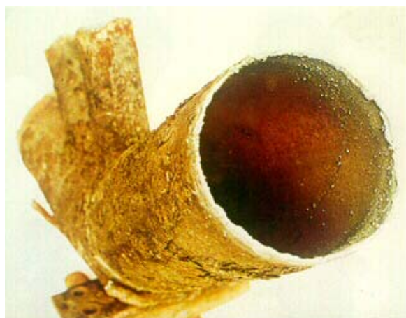
Figure 25: Truss component located over a pickling bath. The external surface shows an advanced state of corrosion, due to the ambient atmosphere, whereas the inside is well preserved, the traces of damage are entirely due to the oxyacetylene cutting operation.
