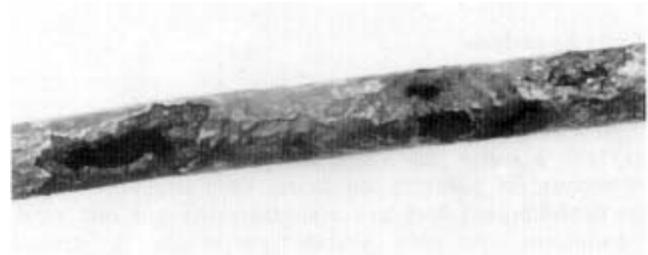
Figure 8: Detail of the corroded openings of the members in fig. 7.
