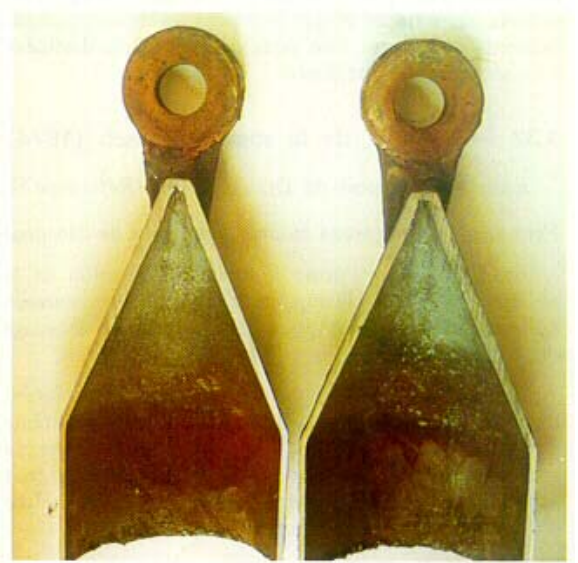
Figure 23: View of the internal faces of the brace component no. 3.
