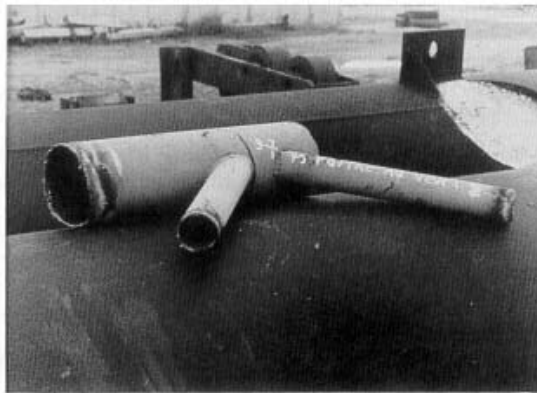
Figure 48: Wind girder 3. Sample removed.
