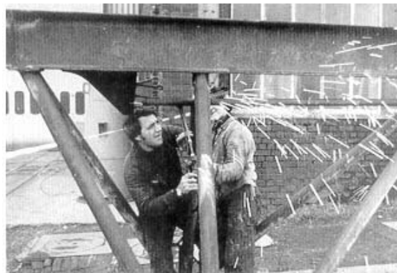
Figure 32 - Cutting out of a sample
