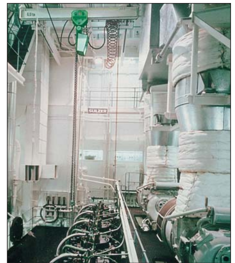
For use in the ship engine room: JDN-PROFI 6 TI in a hand chain trolley.
