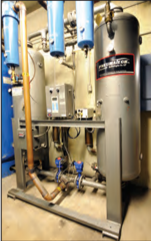
PNEUMATECH PH-750 regenerative air dryer
