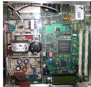
Figure 3-52 Installing FSC300 in FIT500
