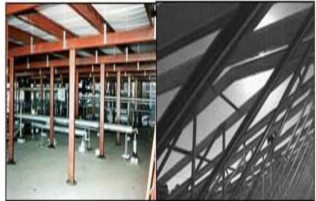
Figure 19-8 Roof Inspections Should Begin Inside the Building
