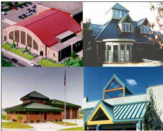
Figure 10-1 The Use and Variety of Metal Roof Designs Are Appealing
