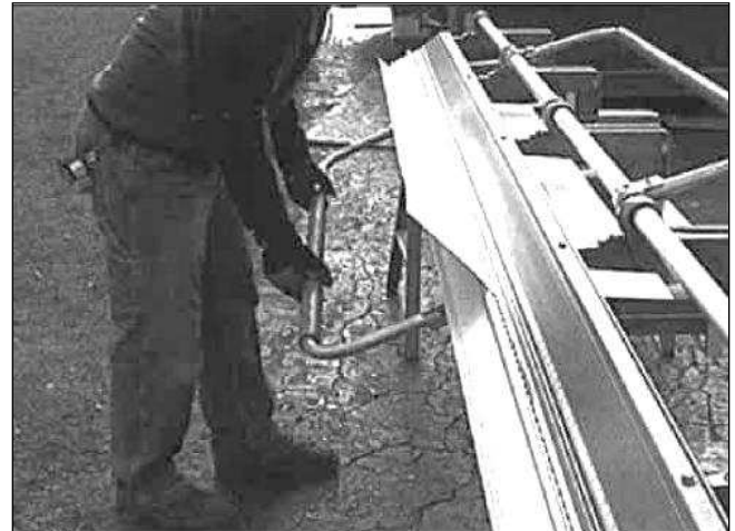
Figure 16-30 On-Site Brake Forming of Roof Material
