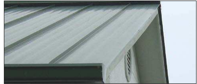
Figure 4-17 Architectural Panel Roof System
