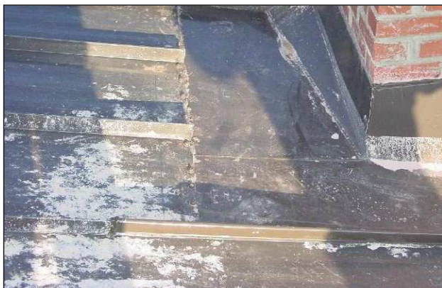
Figure 17-4 Mortar Droppings Should Be Cleaned Immediately.
