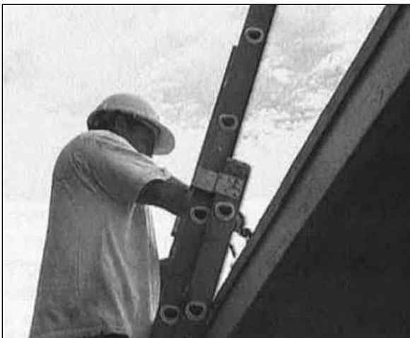
Figure 9-5 Extend the Ladder At Least 3 Feet Above the Eave and Tie It Off
