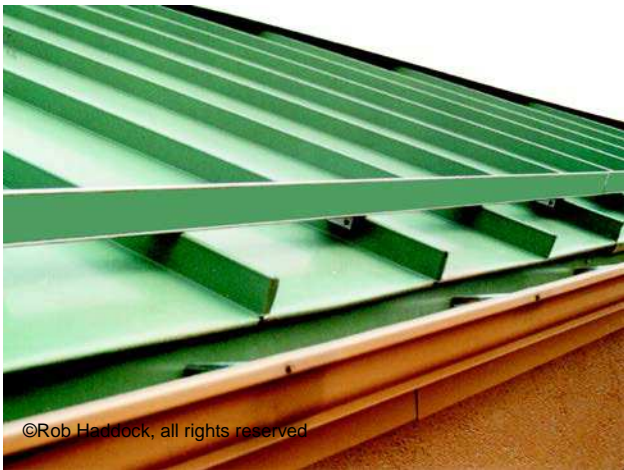
Figure 8-20 A Snow Fence Type Clamp Attached to Standing Seams
