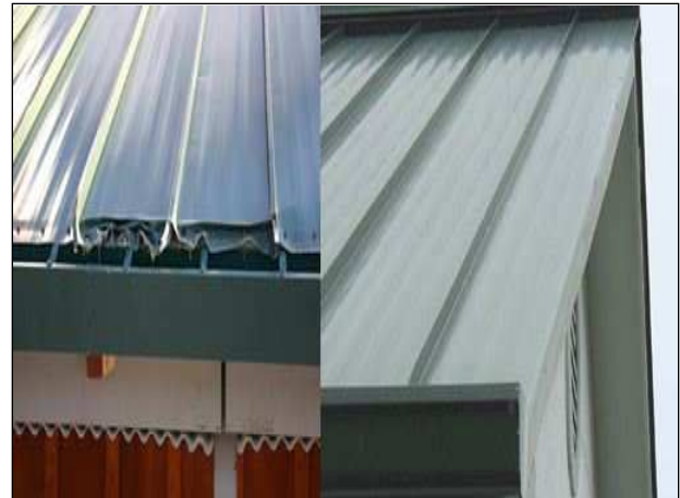
Figure 19-11 Edge and Rake Inspection
