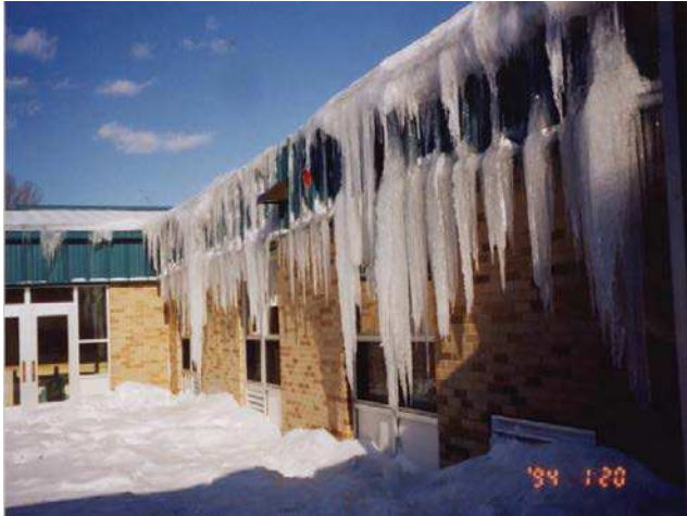
Figure 10-22 Undesirable Ice, Icicles, and Ice Dams
