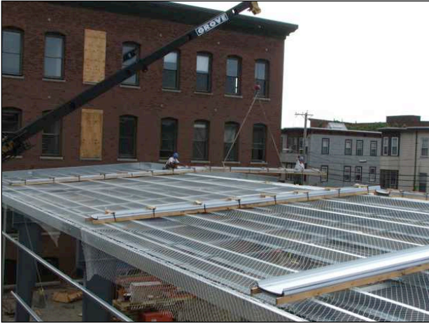
Figure 11-10 Material Should Be Staged at the Bearing Points of the Roof
