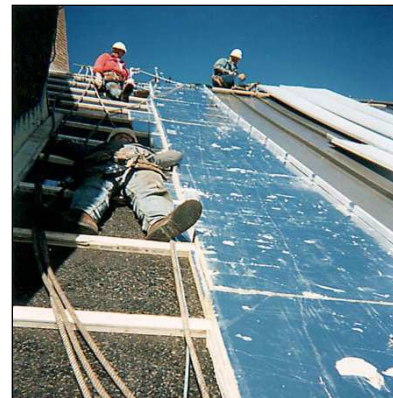
Figure 10-13 Installation of Rigid Polyiso Insulation
