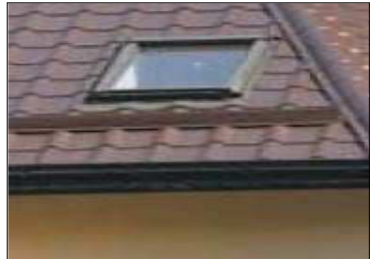
Figure 8-16 Typical Skylight Application
