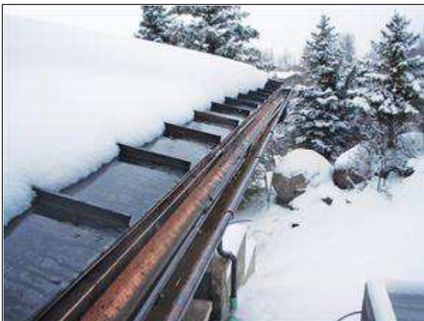
Figure 8-21 Electrical Ice Melt System Installed Along the Fascia Avoids Penetration of the Roof Surface
