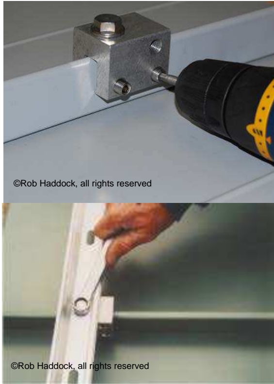
Figure 8-22 Example of Seam Mounted Fence System
