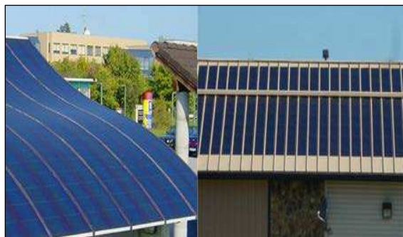
Figure 8-34 Photovoltaic Laminate on a Metal Roof
