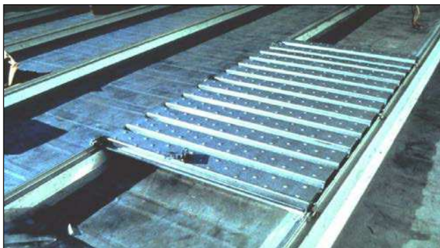
Figure 17-5 Installed Walkway for Heavy Traffic Areas
