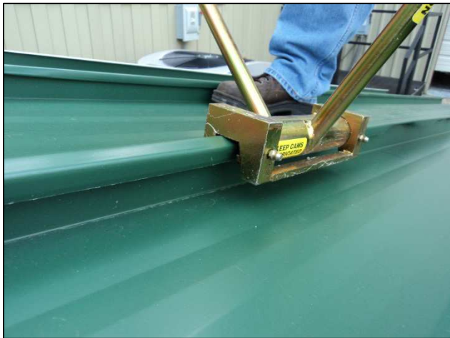
Figure 12-10 Hand-Seamer/Crimper
