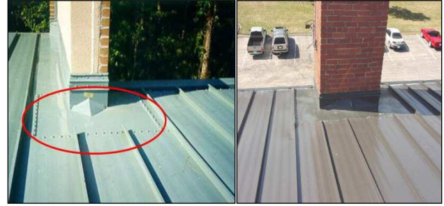
Figure 16-24 Proper Planning Allows Enough Clearance for Runoff
