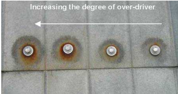
Figure 10-79 Over-Driven Fasteners
