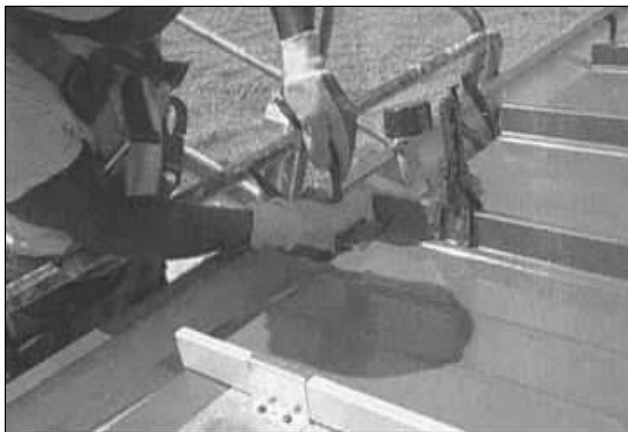
Figure 16-28 Spacer Tools Help Hold Panel Module
