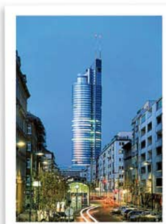
Millenium Tower - 177 access control Wien - AUSTRIA
