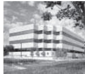
Integrates with Commercial Buildings
