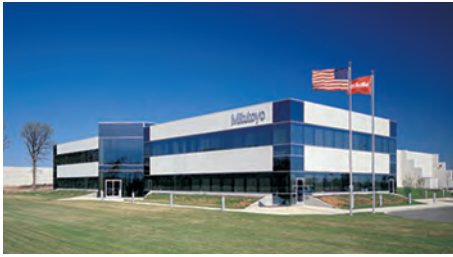
● Mitutoyo America Corporation ■ Corporate Headquarters Aurora, Illinois USA (630) 820-9666
