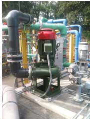
STAR ONE™'s vertical, close-coupled construction and custom-trimmed and fully-enclosed impeller are a few of the proprietary features delivering the industry's longest and most operator-friendly service life.
