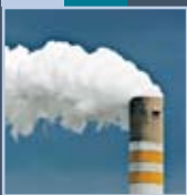
AIR POLLUTION CONTROL
