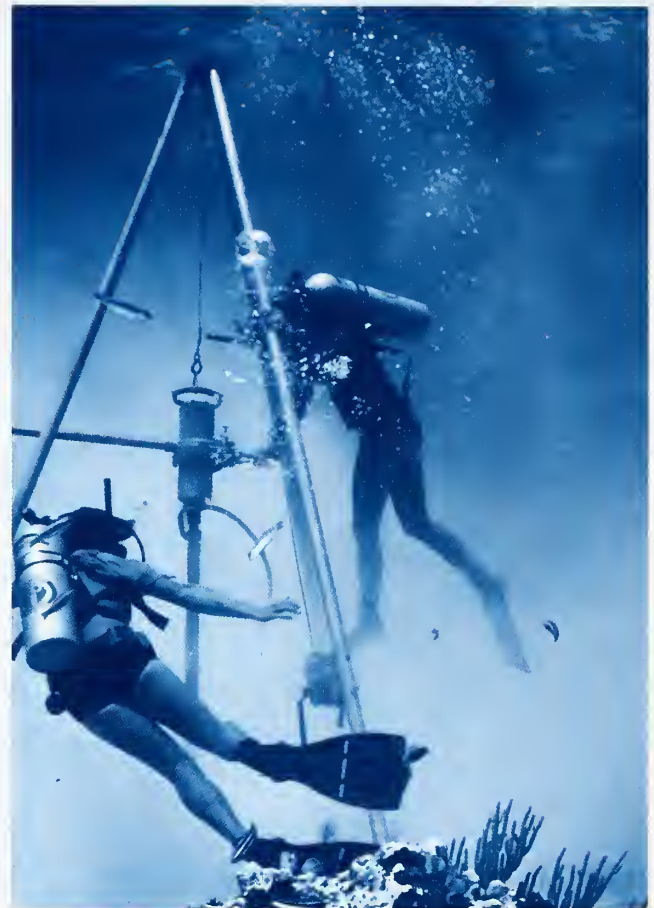
Figure 9-30 Coring in a Deep Reef Environment With a Hydraulic Drill
