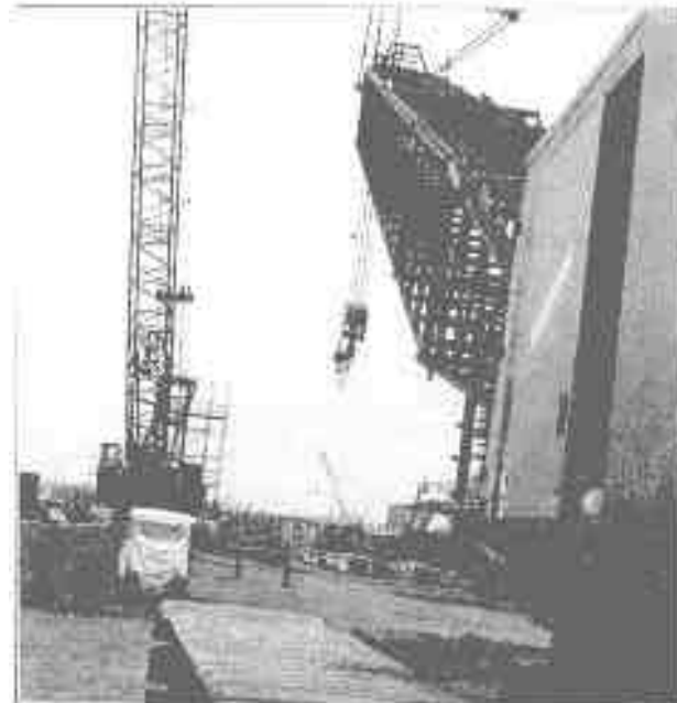
CRAWLER CRANE PREPARED FOR INSPECTION
