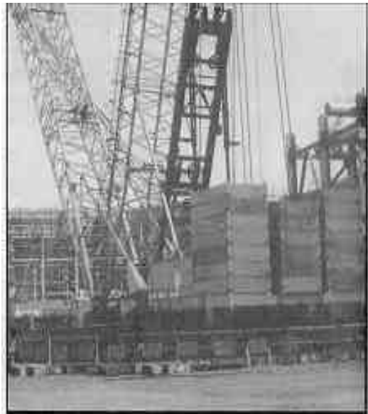
MODERN RINGER CRANE 500 TON CAPACITY
