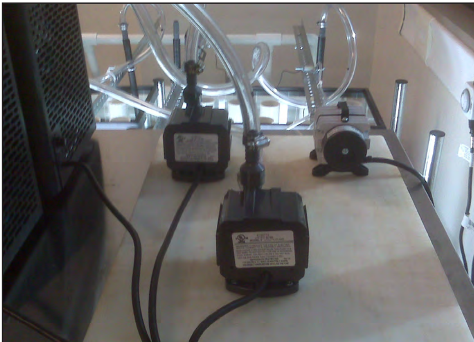
Figure 2.9 Large cutting board used to anchor the chiller and air pumps
