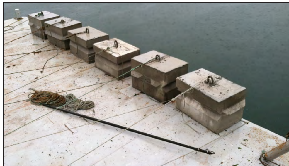
Figure 1.5 Concrete block moorings
