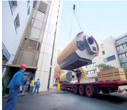
Delivery to site of a Vitomax boiler
