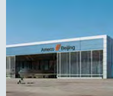
Ameco A380 Hangar Beijing, China
