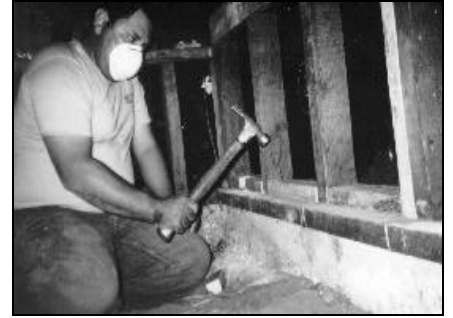
Fig. 3.23 - Cripple Wall Blocking
