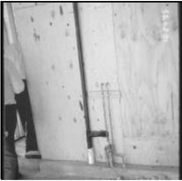
Fig. 3..32-Regulated Penetrations
