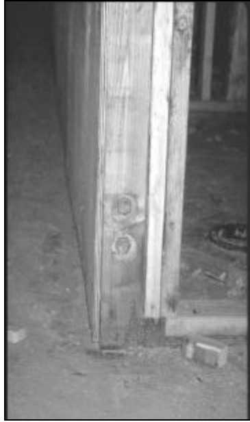
Fig. 3.27 - Too Close to Wall End
