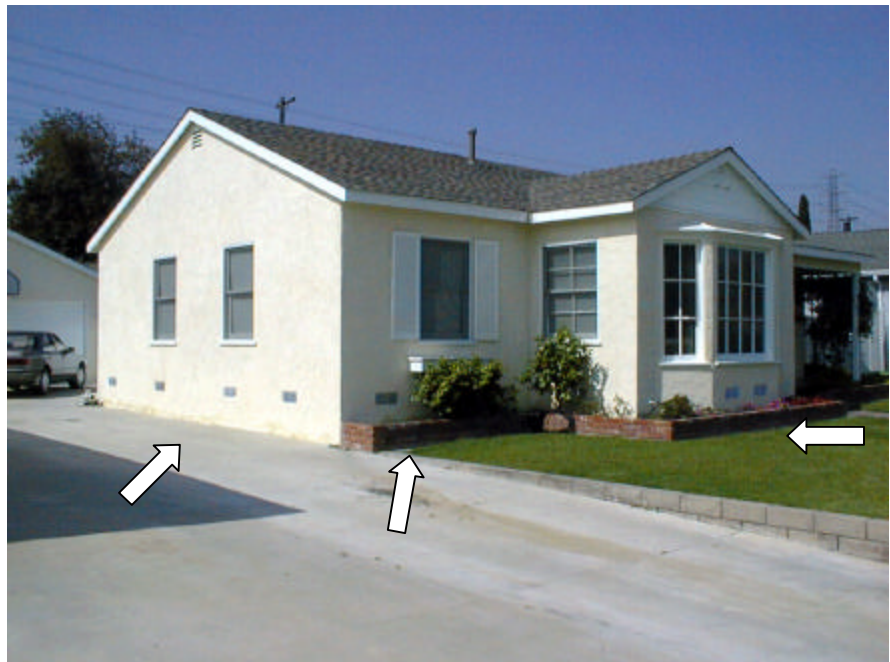
Fig. 3.36 Crawl Space Ventilation
