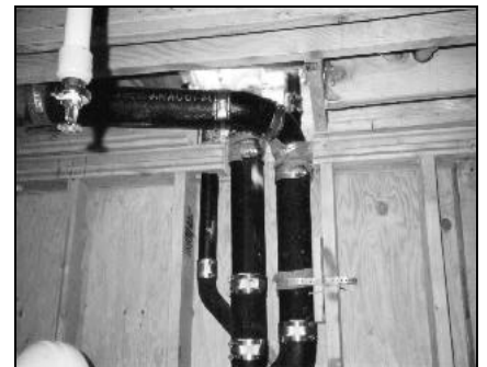
Fig. 3.31 Unregulated Penetrations
