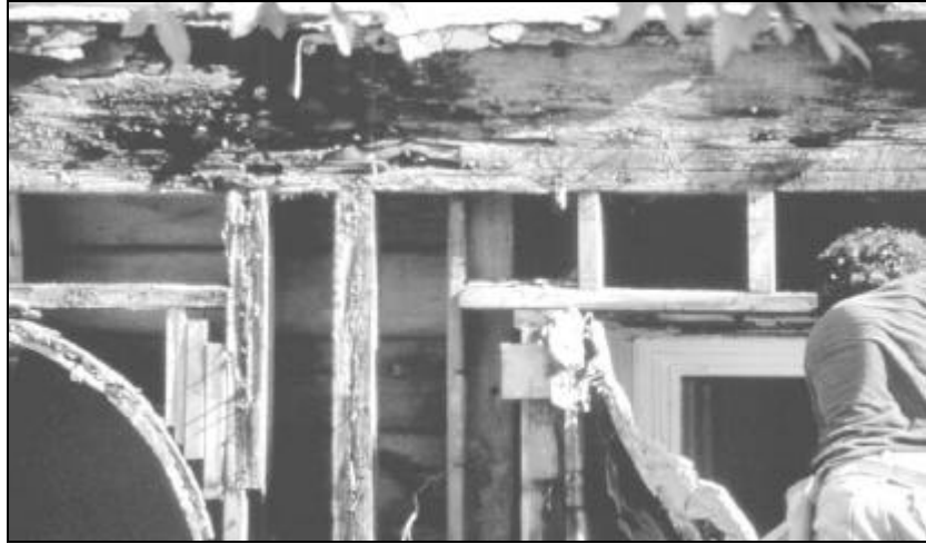
Fig. 3.35 Termite Damage
