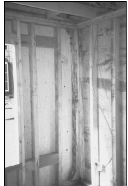
Fig. 3.26 Blocking for Reinforcement
