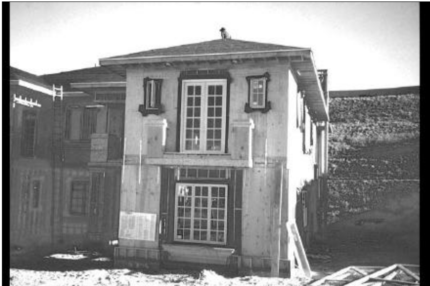
Fig. 3.25 Reinforced Window Openings in Shear Wall
