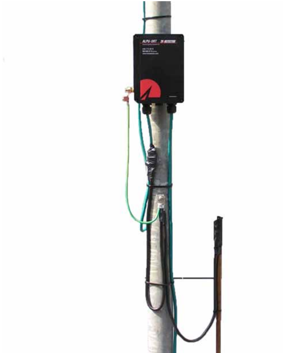
Figure 80 - Lower Grounding Configuration
