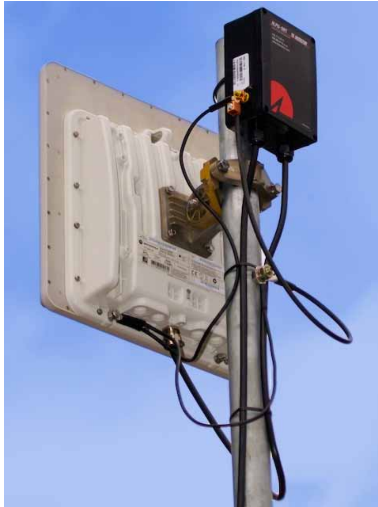
Figure 79 - Upper Grounding Configuration
