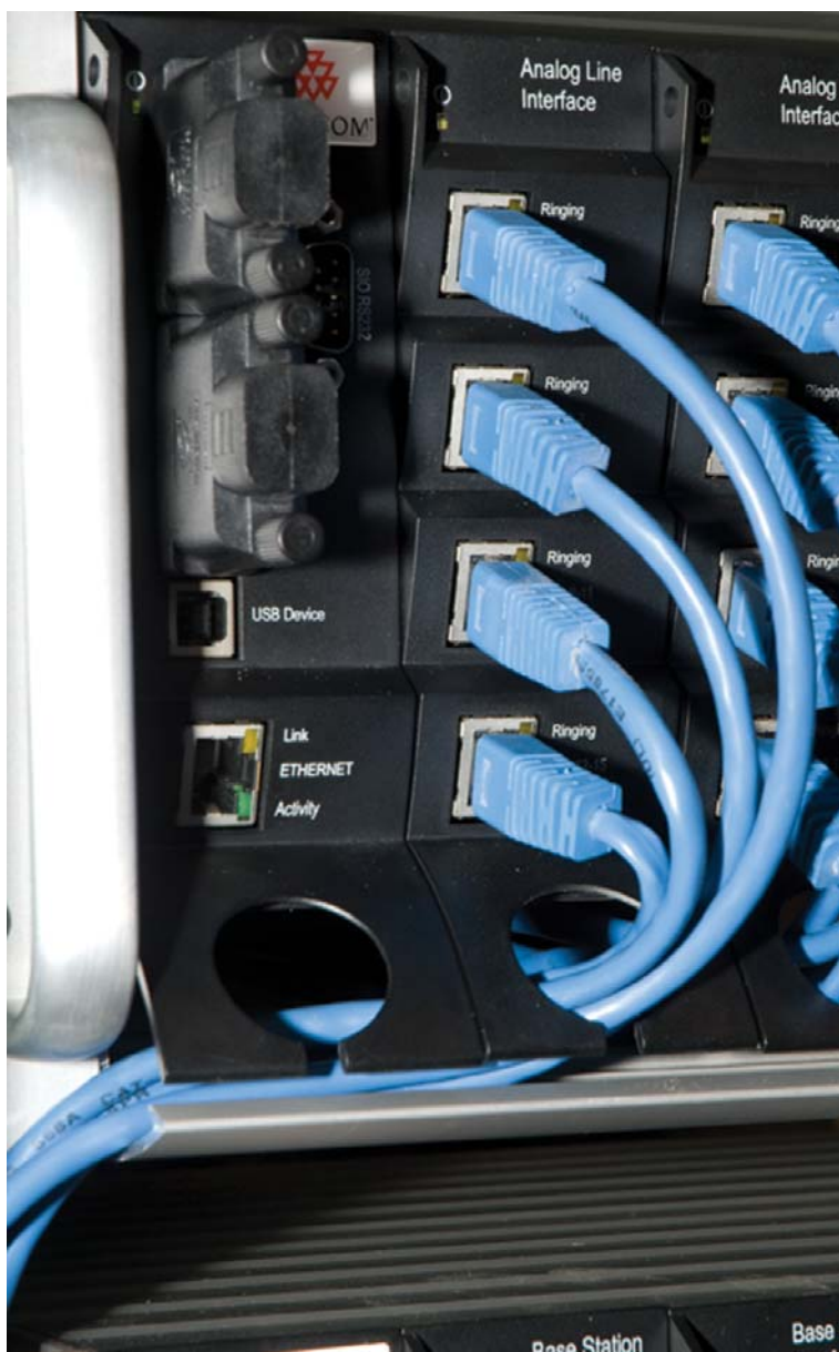
Figure 1-12 Harnessing cables to the side and out.
