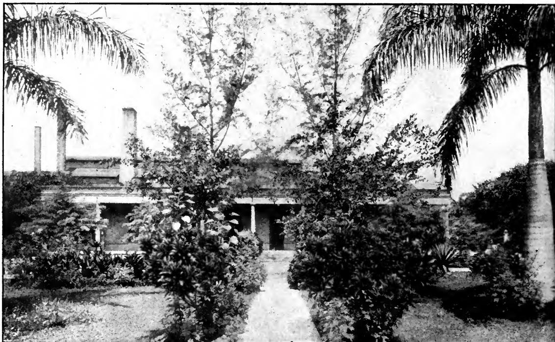
CHRISTMAS DAY AT THE HOME OF 6KW Office building at the Tuinucu Sugar Company plantation
