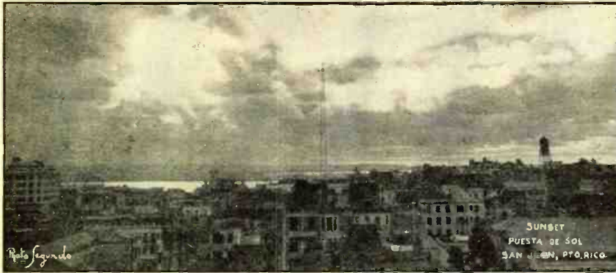
PUERTO RICAN WNEL, 1290 KC., 5 KW. At the left is a "shot" of San Juan, Puerto Rico, with WNEL's mast towering above its surroundings. Photo submitted through courtesy of Observer Johnson, of Chisholm, Minnesota.
