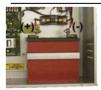
Fig. 8 Battery and 60 amp fuse
