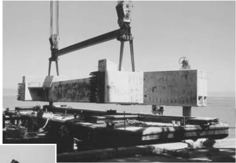
517 ton Bridge Retrofit
