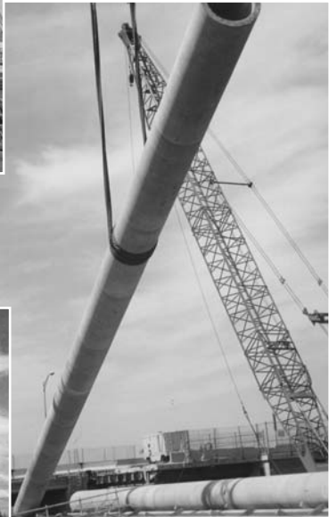
80 ton Concrete Piling
