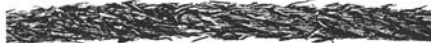
TOO LONG IN SERVICE. Repeated winding and overwinding of this rope on a drum while it was under heavy stress caused the unusually severe wear shown.
