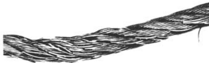
UNDERSIZE SHEAVE GROOVES. Sheaves were too small, causing strands to pinch. Wires then fail in the valley between the strands.
