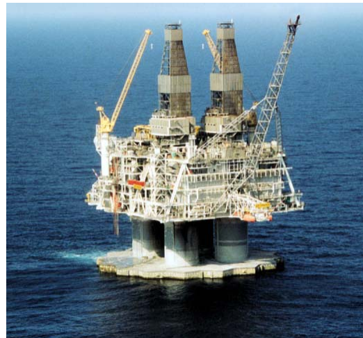
4 LM2500 units, 1994 Hibernia Platform, Nfld
