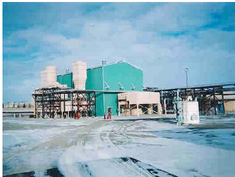
Interpipe Cochrane AB (ANG) Two RB211 GTCHP units
