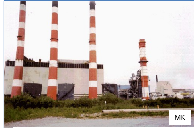
Bayside 285 MW, Saint John NB (Alstom GT24 repowers Courtney Bay oil-fired steam turbine in 2001, NB Power)
