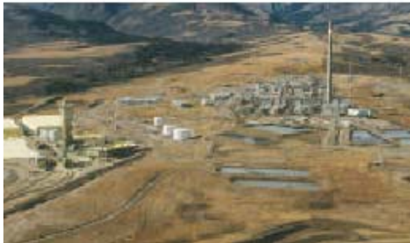
First large Canadian CHP with Aeroderivative GT, (RB211) 1978
