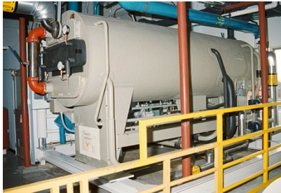
ABSORPTION CHILLER – 200 Tons
