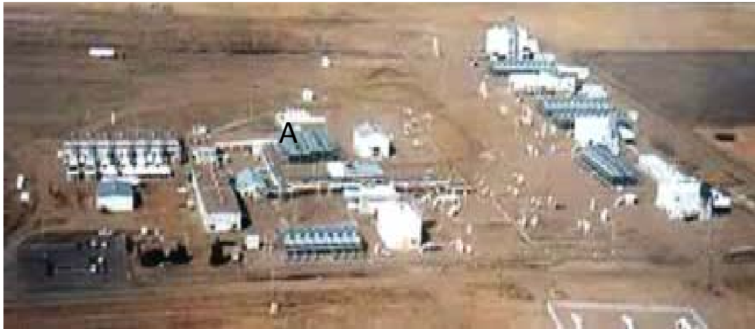
RR Avon, 3 RB211s 2 GE LM2500 (Total 143 MW)
