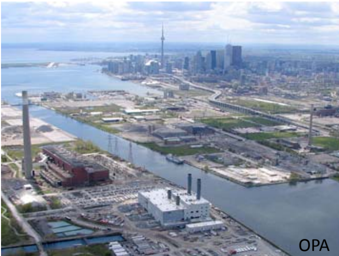
TCPL Portlands , Toronto 550 MW, 2008 (2 GE Frame 7F replace RL. Hearn Stn.)
