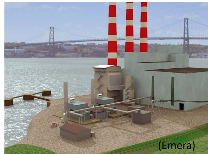
Tufts Cove Emera NSP, Dartmouth, NS Two GE LM6000, with IST OTSGs added in 2009
