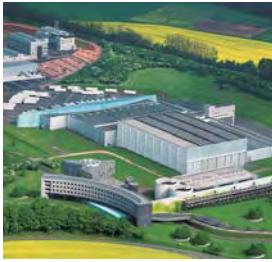
L.I.F.E. pharmaceutical plant B. Braun Melsungen AG: Two Vitomax 200-HS high pressure steam boilers deliver up to 40 t/h for the production of infusion solutions
