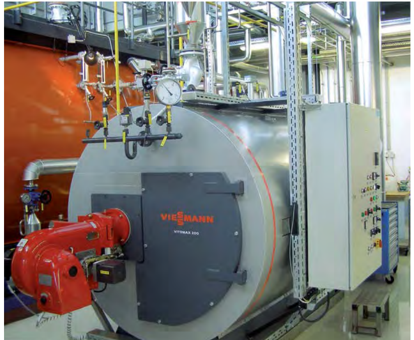
Vitomax 200-HS, type M237 with boiler equipment
