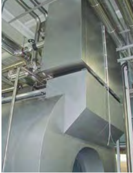
Economiser fitted on a Vitomax 200-HS
