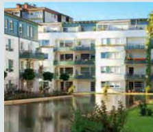
"Wohnoase" residential park in Regensburg, Germany
