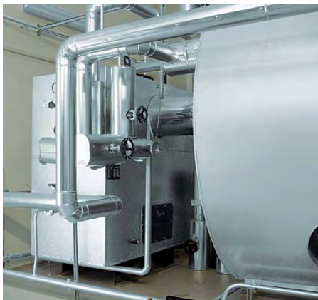
Vitomax 200-HS steam boiler with downstream economiser
