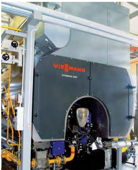
Vitomax 200-HS steam boiler with superheater
