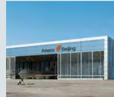
Ameco A380 Hangar Beijing, China
