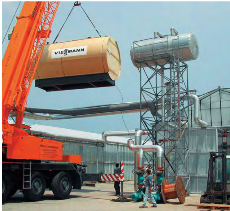
Installing the Vitomax by mobile crane
