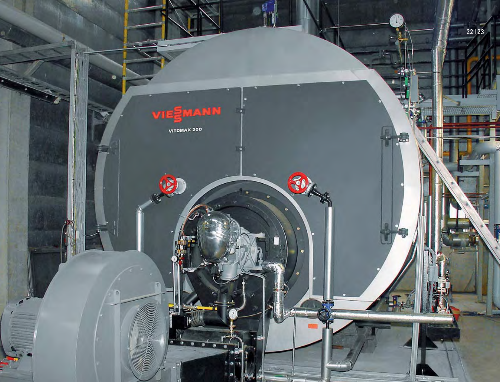
Special version of the Vitomax 200-HS steam boiler for burning animal fat
