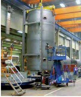
Welding the pressure vessel in the optimum welding position
