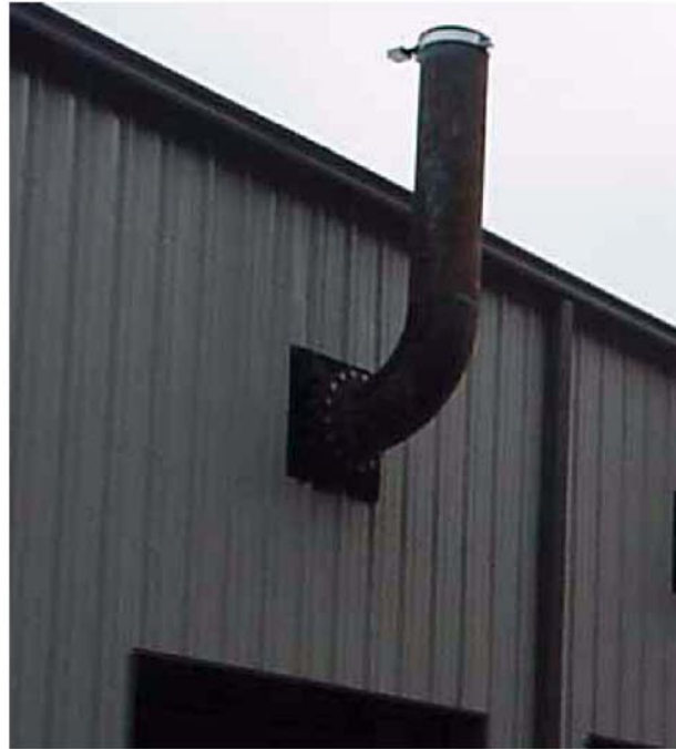
FIGURE 57. A SIMPLE EXHAUST SYSTEM FITTED WITH A RAIN CAP TO PREVENT RAIN FROM ENTERING THE EXHAUST.
