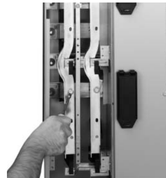
Field Phase Balancing
