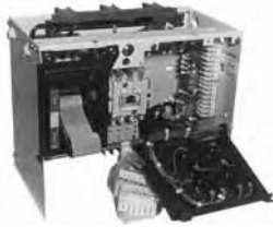
F2100 Replacement Starter Unit (1995 to Present)
