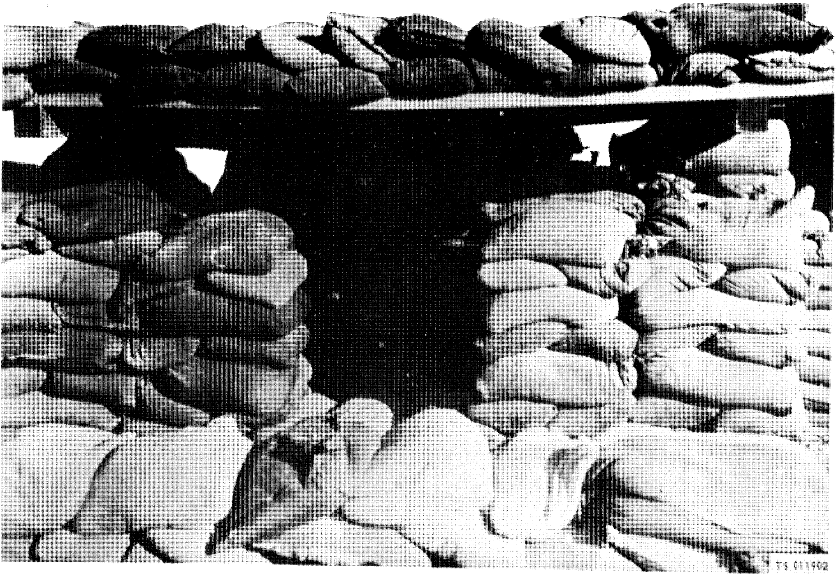
Figure 4-8. Revetment, front view.
