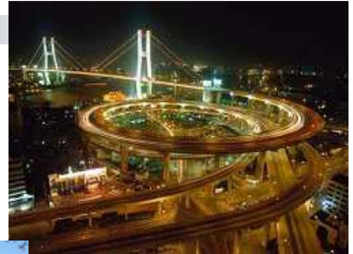
Old Nanpu Bridge (double loop ramp), Shanghai,
