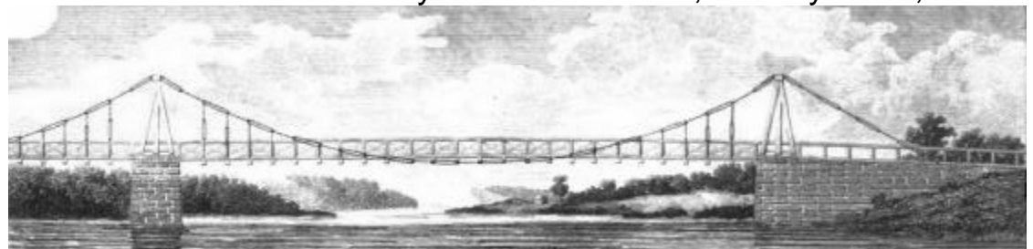
First modern suspension bridge -James Finley's -Jacob's Creek, Pennsylvania, 1801
