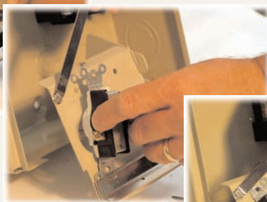
IWC OPENED TO INSTALL WIRING DEVICES
