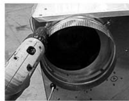
Figure 4: Installing exhaust collar.
