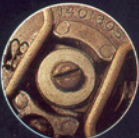
High-radioactivity equipment inside nuclear reactor as seen through Lenox sectional borescope with radiation-resistant lenses.
