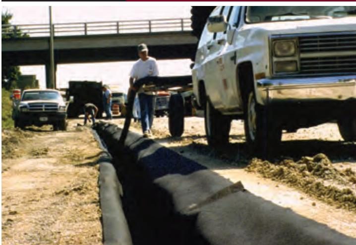
This is one of the most common applications of geotextiles in the construction of roadways, landfills, athletic fields etc, allowing for rapid removal of water or other fluids while providing excellent soil retention, assuring long-term free flowing drainage.
