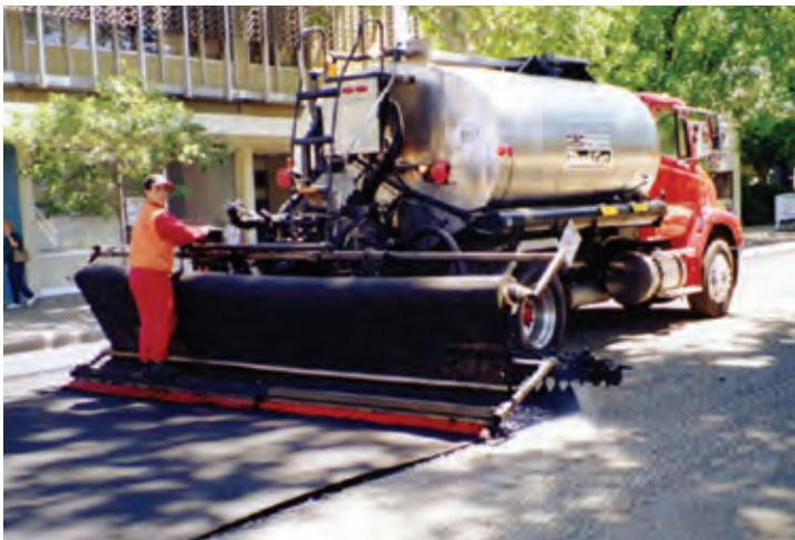
Asphalt overlay fabrics can extend the life of all existing paved areas. These specially manufactured nonwoven geotextiles are first saturated with heated liquid asphalt during installation, and creates a moisture barrier between old and new pavement. In addition, they absorb stresses to retard reflective cracking, thereby improving and extending the overall performance of the new overlay.
