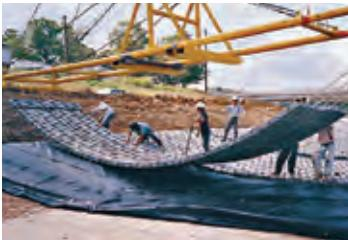
These were the very first applications of a geotextile in 1958. The fabric, which lies beneath various forms of riprap cover (i.e. rock, gabions and mattresses, concrete pattern-placed units, etc.), allows for free drainage of water while holding back fines thereby preventing shoreline and other erosion.
