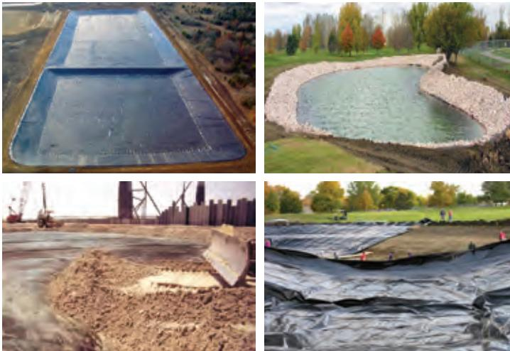
Containment projects utilize a wide variety of geosynthetics for veneer reinforcement, geomembrane protection, drainage, steepened slopes, vegetation/erosion control, gas venting and capping/closures.
