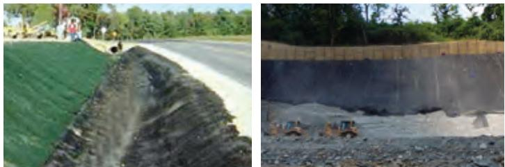
(1978-1979) Carthage Mills works with the USACOE for development of the *first* effective Design Criteria for Fabric-Reinforced Embankments on Soft Soil. –Pinto Pass Mobile, AL.
