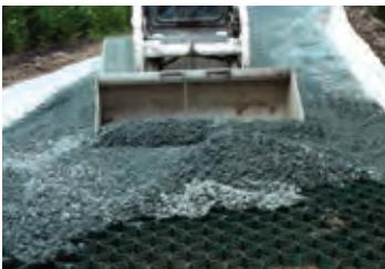
For low cost, geosynthetics can significantly extend the life of everyday structures by preventing the intermixing of subgrade soils and the aggregate base, and/or stabilizing poor subgrades.
