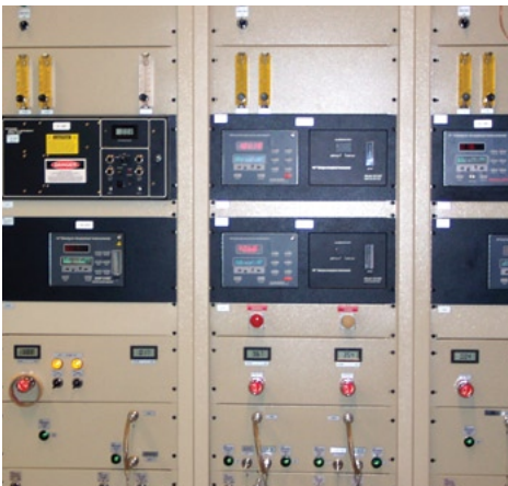
Medical gas racks per US and European Pharmacopoeia regulations
