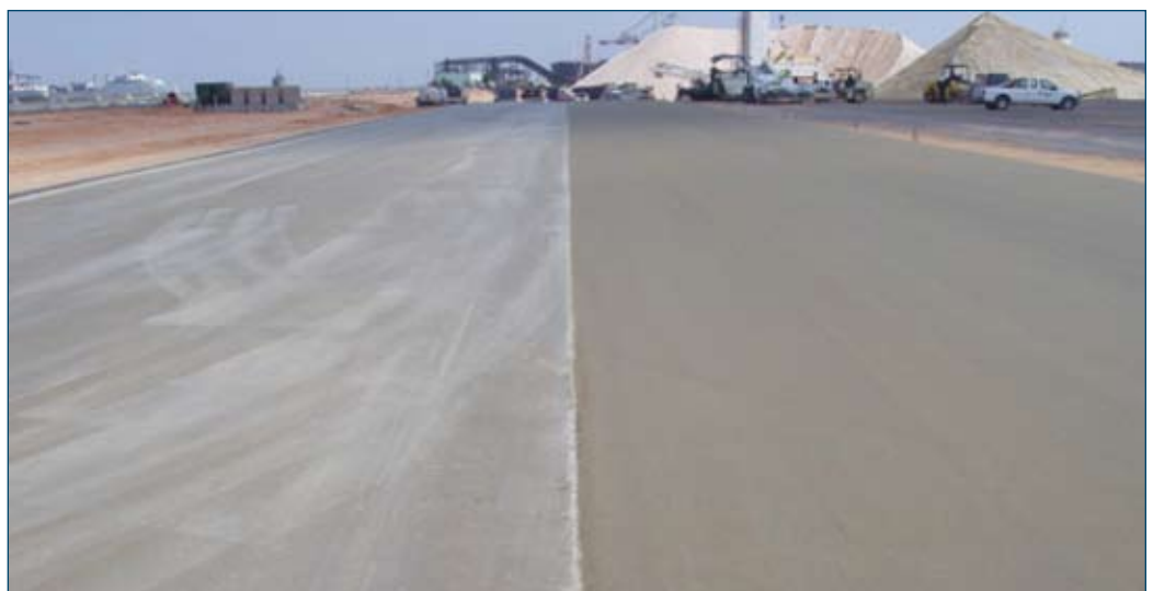
Figure 7-14. Longitudinal construction joint
