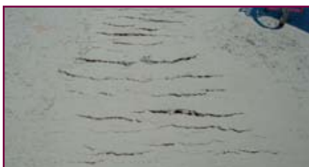
Minor tearing of the mix from rolling
