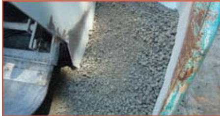
Segregation in paving hopper
