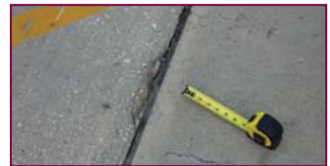
Spalling at cold joint
