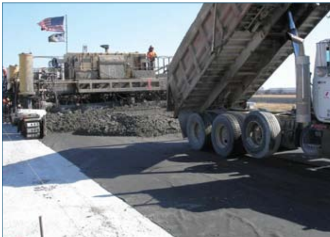
Figure 2-7. Concrete paving with geotextile fabric layer
