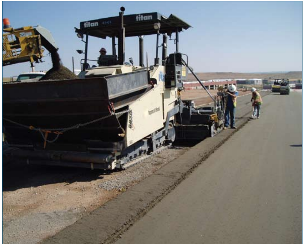
Figure 7-6. Fresh longitudinal joint
