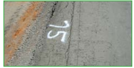
Required target density is not achieved
