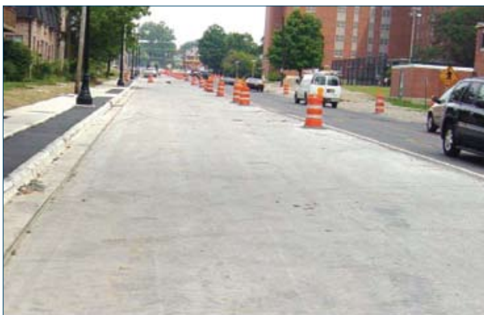
Figure 2-4. RCC pavement constructed on an arterial street in Columbus, Ohio
