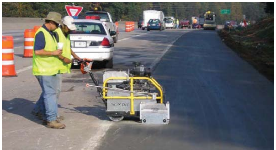
Figure 7-13. Shoulder transverse sawed joint
