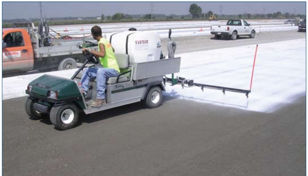
Figure 7-16. Application of curing compound
