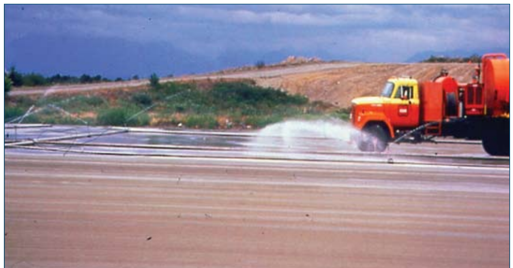
Figure 7-17. Moisture curing using sprinklers and fog spraying
