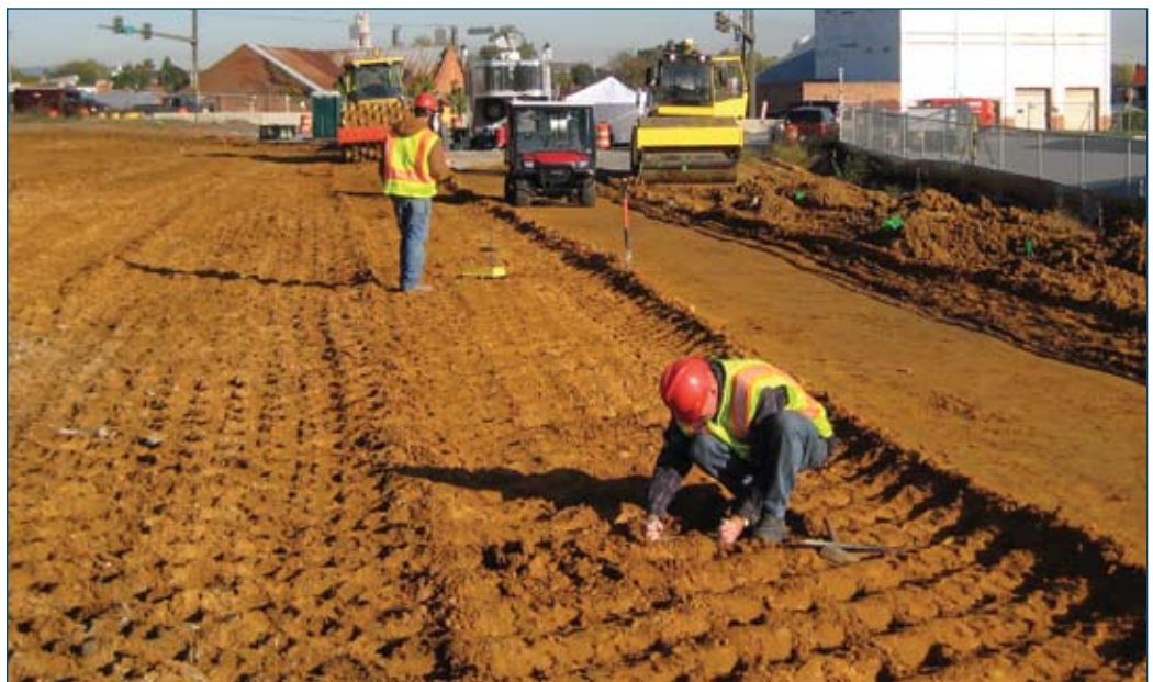
Figure 7-1. Preparation of subgrade
