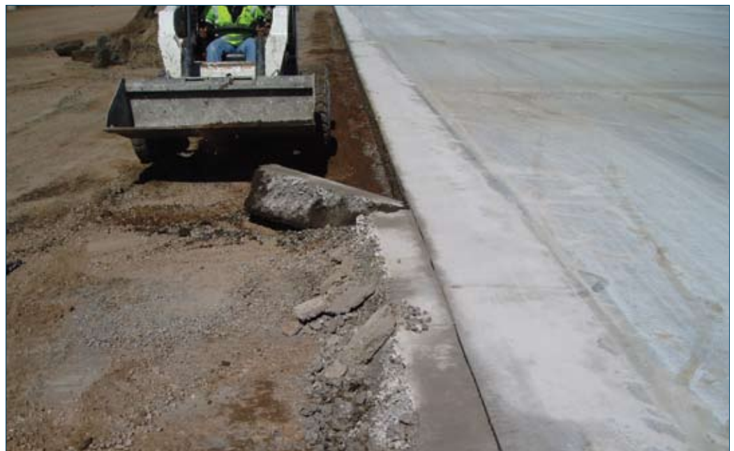
Figure 7-7. Finished longitudinal construction cold joint
