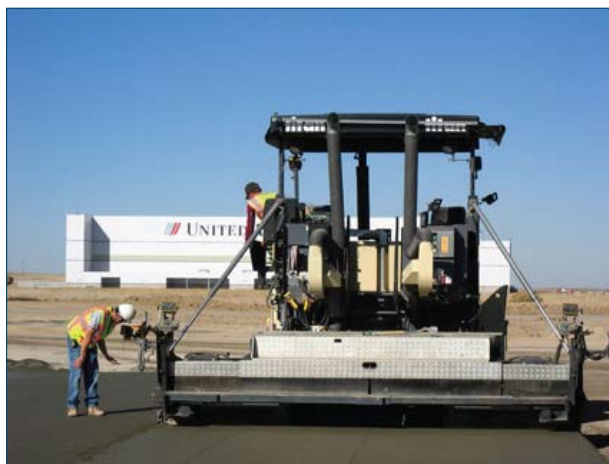
Figure 2-3. RCC paving operation at an airport
