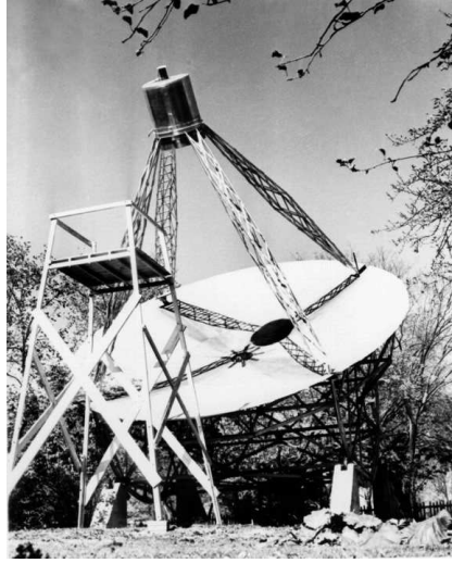
Figure 1.1: First steerable radio telescope, constructed by Grote Reber. Image courtesy of NRAO/AUI.
