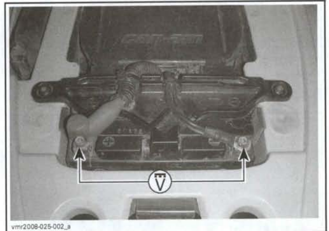
BATTERY VOLTAGE TEST (NO LOAD)
