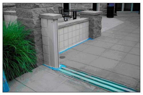
Figure 5-6. The City of Boulder, Colorado, installed a "pop up" closure to this floodwall at a City office building subject to flash floods. The closure floats up into place automatically when the site is flooded.
