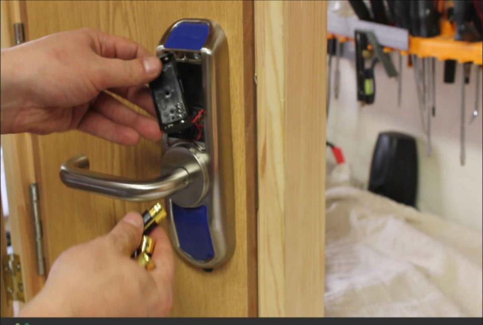
Install AA batteries ensuring correct polarity.
