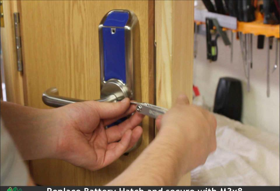
Replace Battery Hatch and secure with M3x8 screw.
