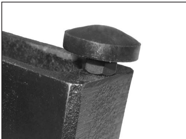
Figure 37. Installed rail pad.
